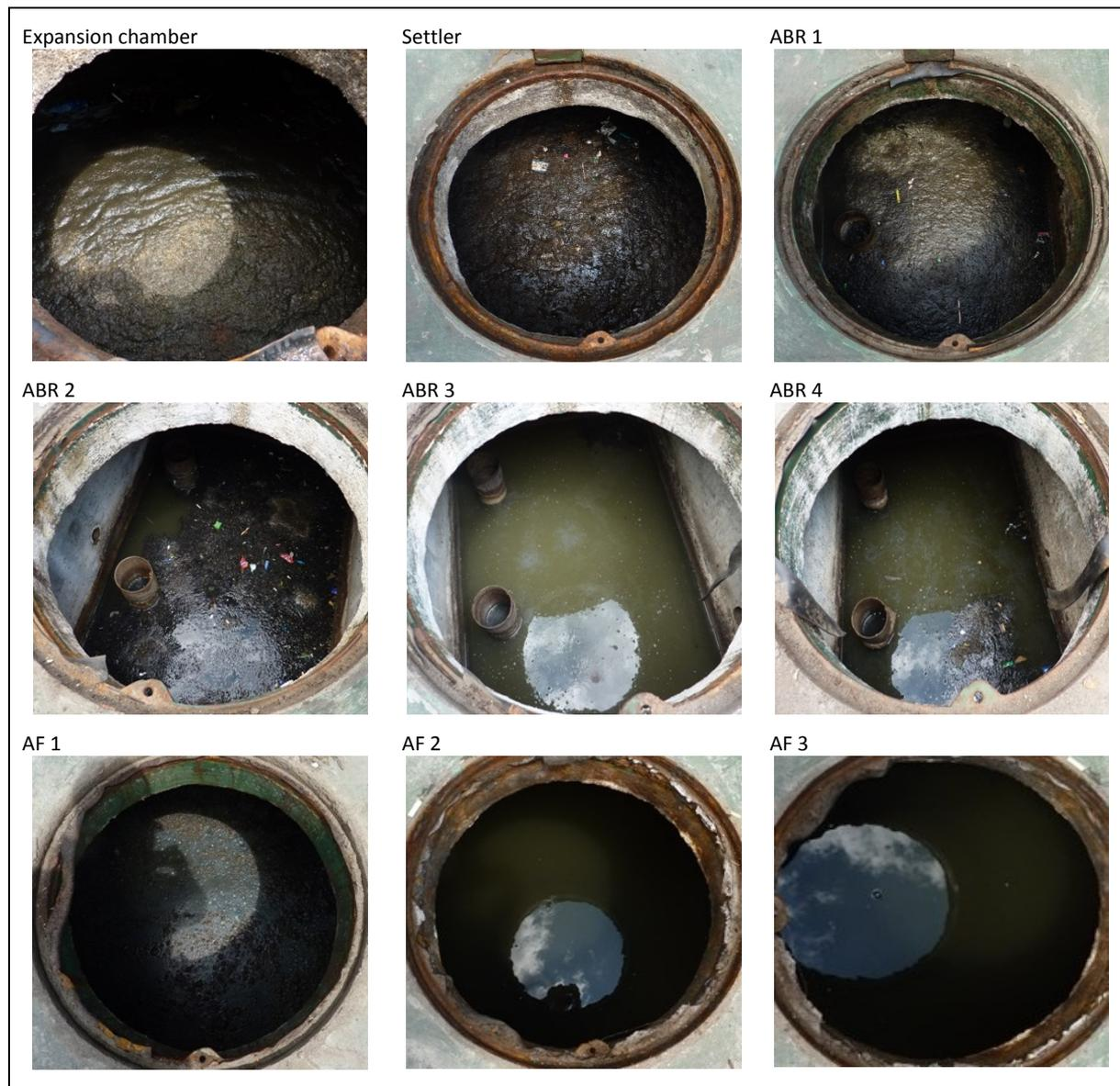
Figure 84: Settler, ABR and AF chamber supernatants as photographed on 02.09.2013
