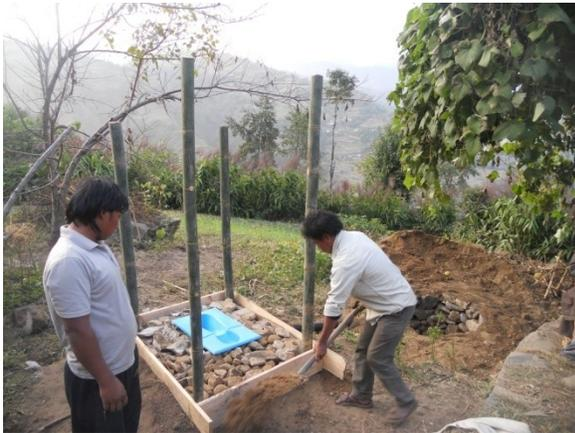
The photo shows a typical low cost toilet that the villagers were trained to construct. It can be built in a day. Wall, door and roof can be built after casting the vertical poles in the concrete. It costs less than the traditional one. However people did not like it very much because they prefer a strong and thick masonry wall.
