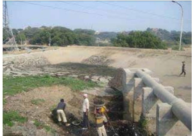
Figure 2.16 Desludging of anaerobic pond (Source: Kazmi 2003)
