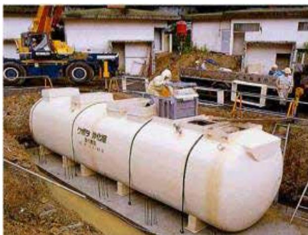
Fig. 2.32: A Typical Package Contact Aeration System
