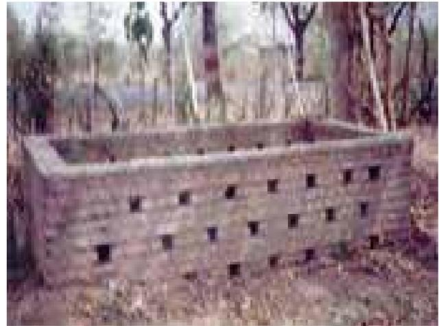
Fig. 3.3 A NADEP composting showing aeration
