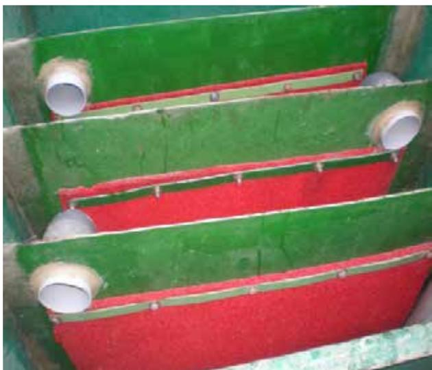
Fig. 2.4 DRDO Biotanks showing different chambers
