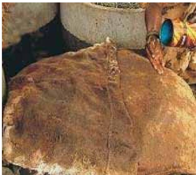
Fig 3.6. Concrete ring cover with gunny bag
