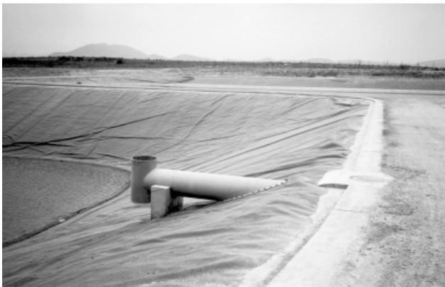
Fig.2.17 Covering of base of pond with plastic sheet Source- (Duncan Mara 1997)
