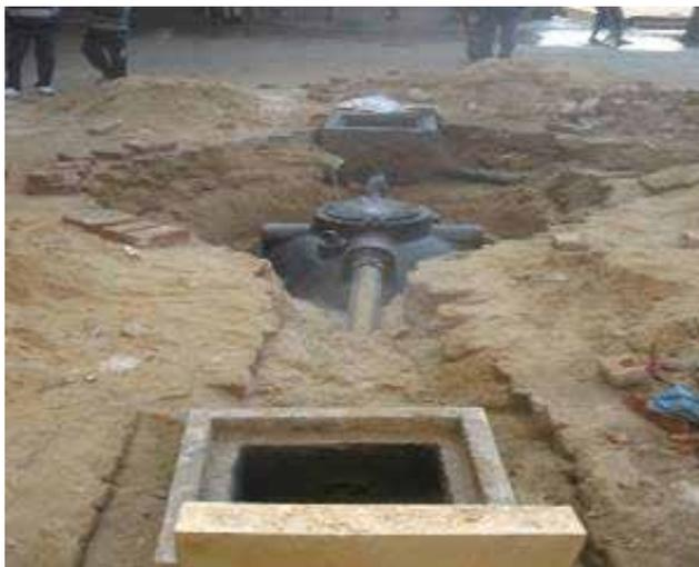
**Figure 2.10: A prefabricated Anaerobic Filter installed under Sponsored Project by MDWS**
