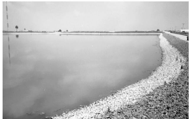
Fig.2.18 A WSP pond with boulders at the base of embankment. Source- (Duncan Mara 1997)
