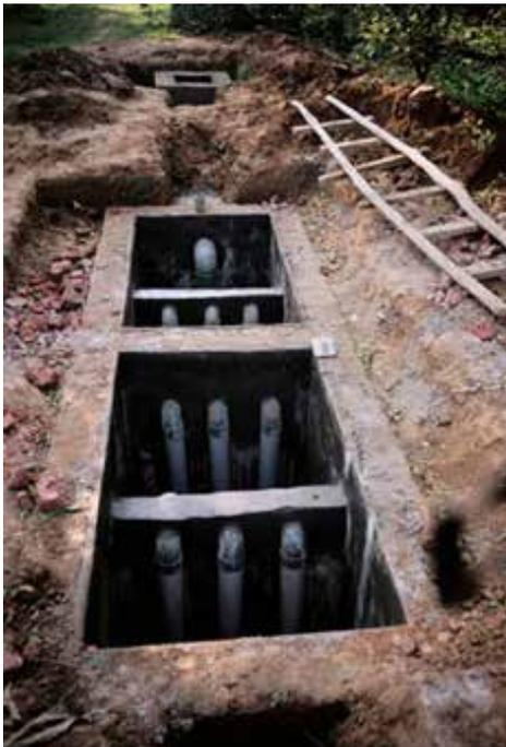
Fig. 2.29: An ABR under construction
