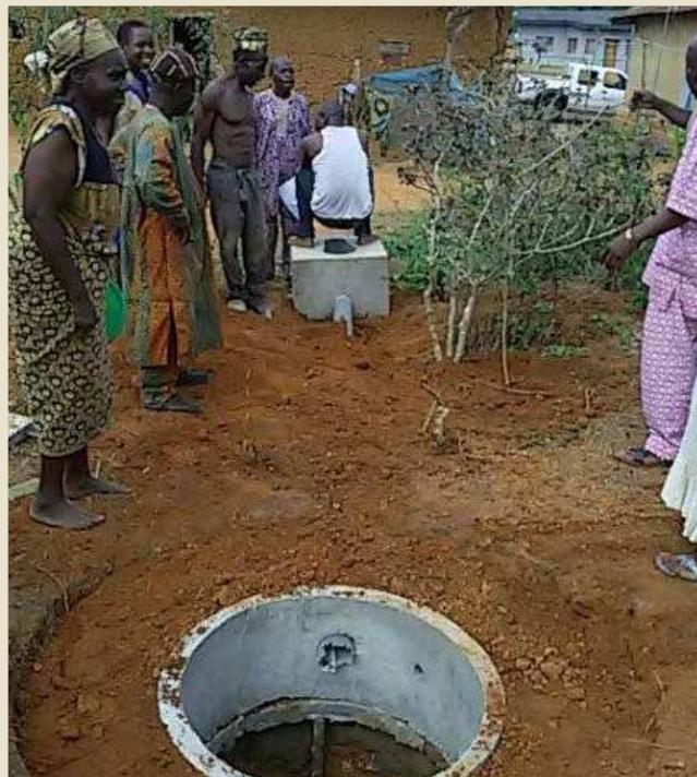
*A pour-flush latrine with offset pit under construction.*
