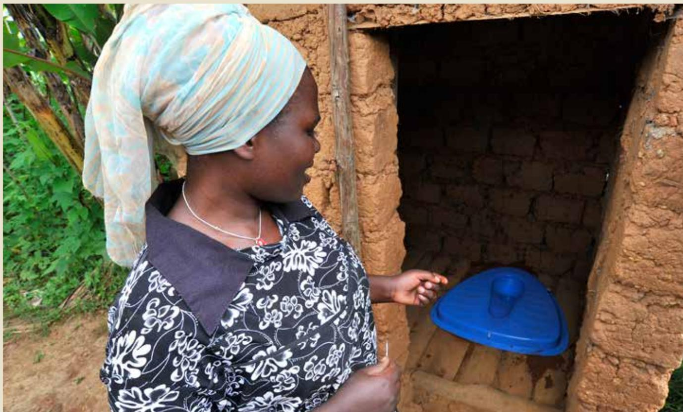
*A prototype of the new American Standard plastic slab with SaTo pan fitted in an existing latrine in Rwanda.*
