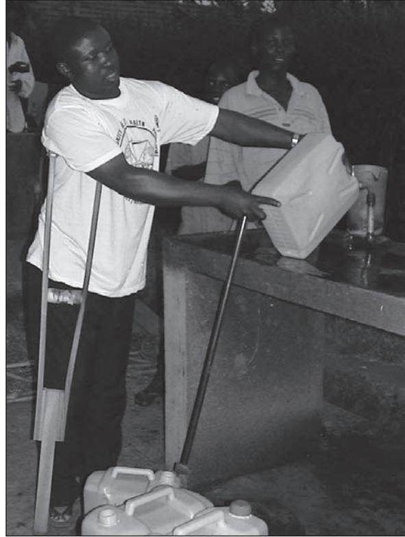
Figure 6.17. Taps ~25cm above a concrete shelf (H: ~1m) do not require the user to bend.
