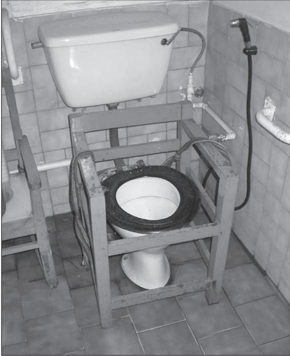
Figure 7.12. Painted wooden frame around pedestal toilet seat.
