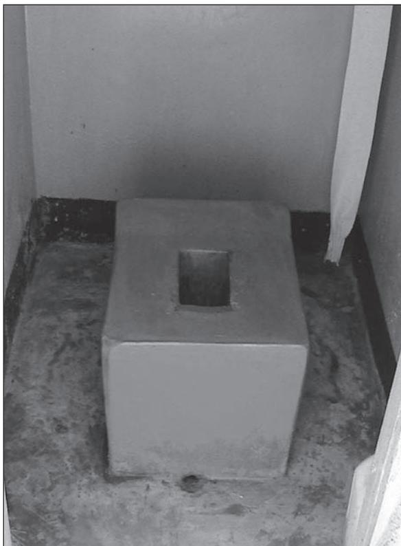
Figure 7.24. Toilet seat made of bricks, plastered with cement mortar and painted. Raised at the back for extra support.
