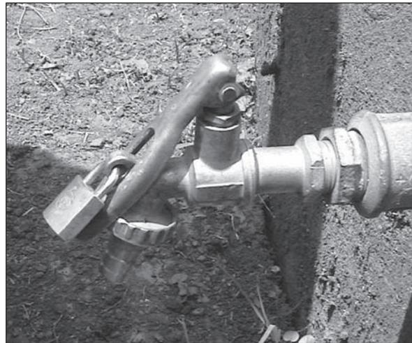
Figure 6.22. Lever operated tap with padlock. Unsuitable for a person with limited grip or stiff fingers.
