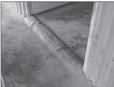
Figure 9.24. Flood prevention threshold has been rounded for easier wheelchair access.
