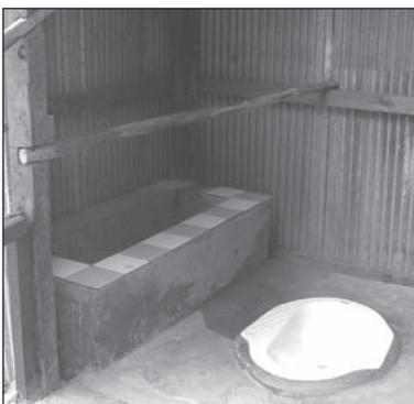
Figure 9.95. Wooden handrail from door to back wall of toilet.
