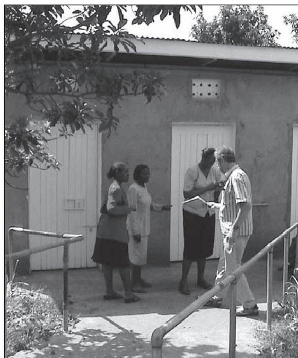
Figure 5.10. Wide concrete ramp with handrails both sides.
