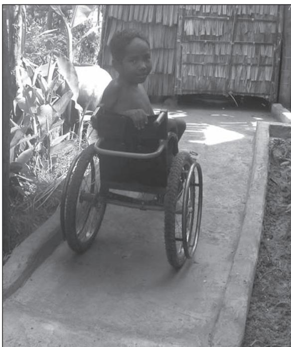
Figure 5.9. Concrete ramp from house to bathing area and toilet.
