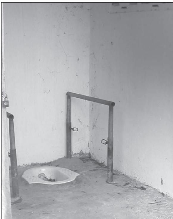
Figure 7.43. Squat toilet installed level with the surrounding floor.
