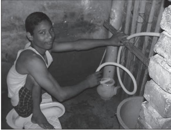
Figure 7.8. Horizontal wooden bar tied to existing pipes in front of toilet. H of bar (~70cm) was decided by user. No choice of distance for bar – nearer would be more comfortable. (Case-study 9.6, page 177)
