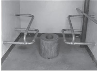
Figure 9.124. Raised toilet seat with handrails for support.
