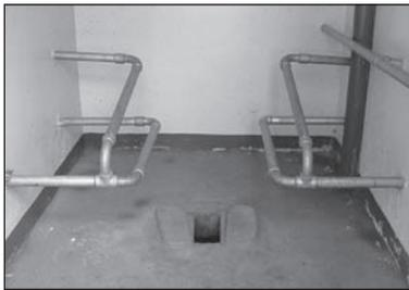
Figure 9.125. Squat latrine with handrails for support.
