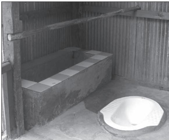
Figure 7.53. Water trough inside toilet cubicle.
