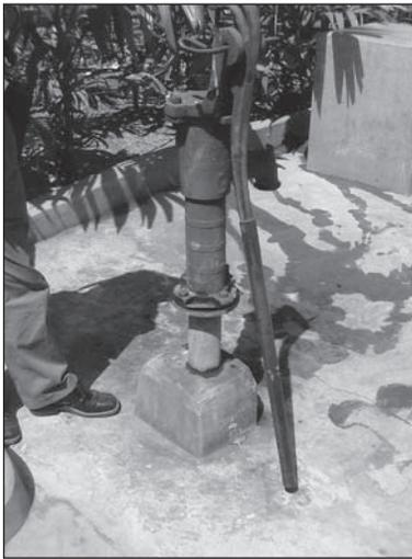
Figure 9.14. Water drains away from the apron.
