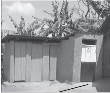
Figure 9.117. Wheelchair accessible toilet on the right. Arrow shows concrete ramp.
