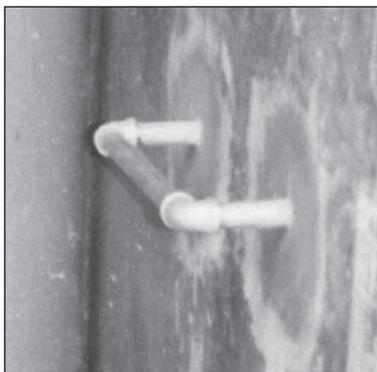
Figure 9.144. Handrail cemented to the wall.
