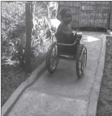
Figure 9.68. Concrete ramp leading to bathing area.
