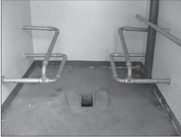
Figure 7.4. Diagonal and horizontal rails fixed to side walls at different heights. Note additional horizontal rail from front to back of wall on the right.
