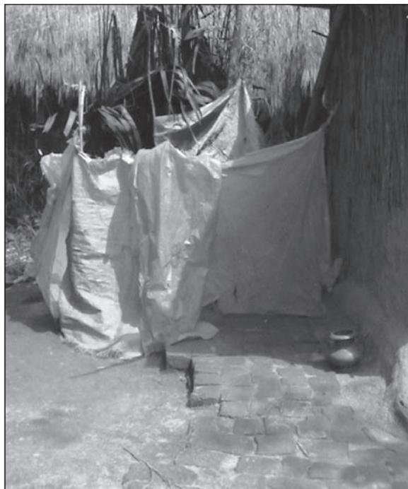
Figure 5.8. Brick path with earth and sand pointing leading to a bathing area.
