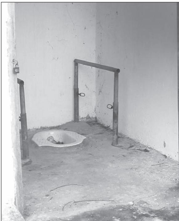
Figure 7.17. Handrails of adjustable height, suitable for a growing child.
