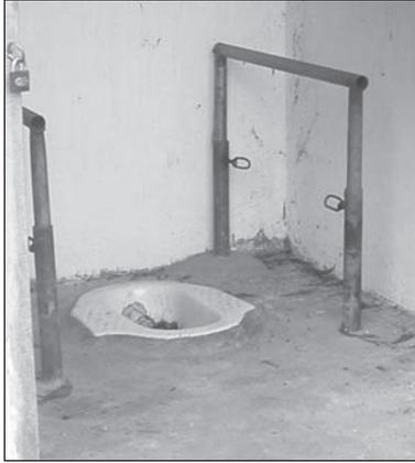
Figure 9.80. Adjustable handrails.
