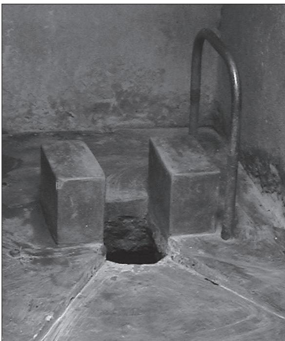
Figure 7.26. Twin cement-plastered brick sitting blocks. Height: 25cm; gap: 14cm. The gap makes anal cleansing easier than on an ordinary seat.
