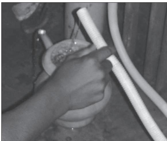
Figure 7.54. Flexible hose attached to a tap allows the user to fill a container with water using only one hand.
