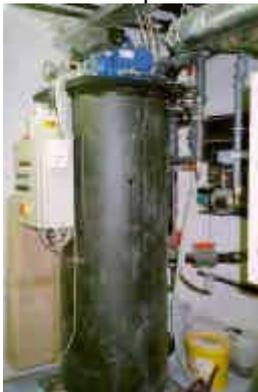
**Figure 3:** Vacuum-system reduces water use for Toilet Flushing in apartment building; before anaerobic treatment, Freiburg, Germany.
