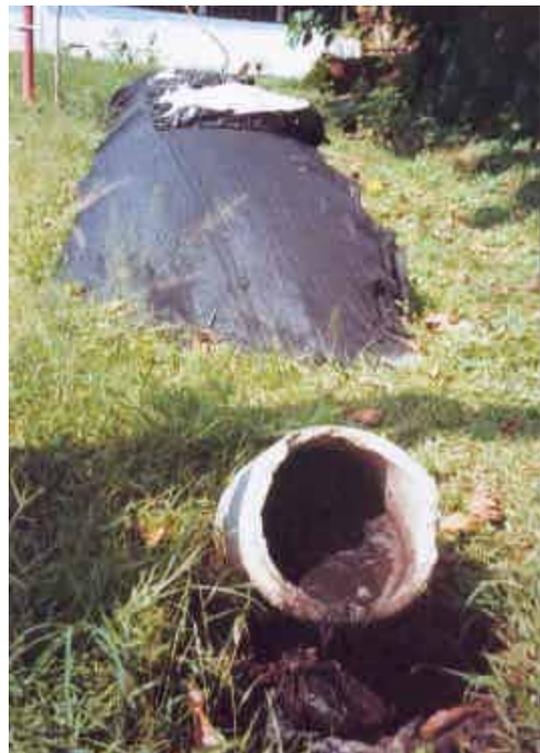
**Figure 6:** A common type of agricultural biogas plant in Cuba consisting of a long plastic tunnel with an in- and outlet made of concrete tubes:
