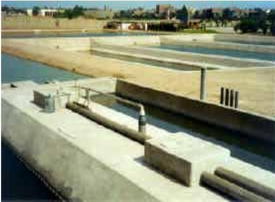
**Figure 1:** Appropriate decentral waste water treatment through a UASB-System in Lima.
