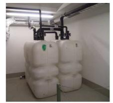
**Fig. 7:** The two plastic urine tanks (currently bypassed) in the school building's basement have a capacity of  $1.5 \text{ m}^3$  each (source: OtterWasser GmbH).
