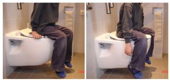
**Fig. 10:** Left: ordinary (problematic) sitting position of a child on a Roediger NoMix toilet. Right: optimal (but less comfortable) sitting position of a child (source: LINZ AG).
