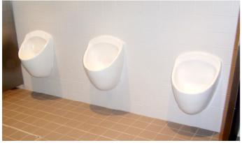
**Fig. 6:** Waterless urinals for boys from the Austrian company Hellbrok in the school building – hung lower than for adults (source: OtterWasser GmbH).
