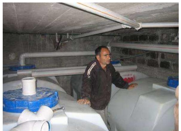
**Fig. 11:** Urine tanks (4 x 2 m<sup>3</sup>) in the basement of the school (source: AWHHE, 2006)
