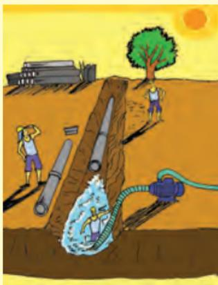
Oozing ground water during excavation should be removed manually or using pumps.
