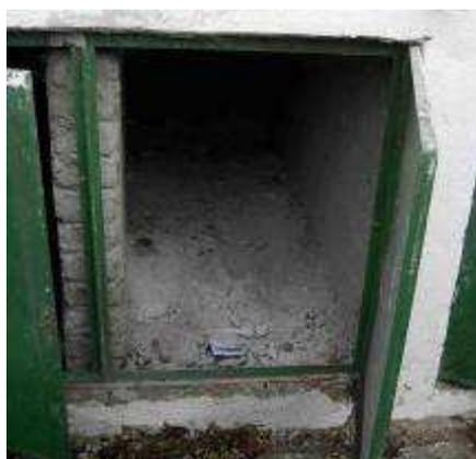
Figure 7: faeces collection chamber (source: WECF)
