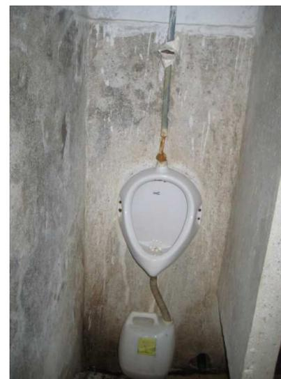
**Fig. 4:** Collection of undiluted fresh human urine from water-flushed standard urinals by blocking water flush during urine collection.
