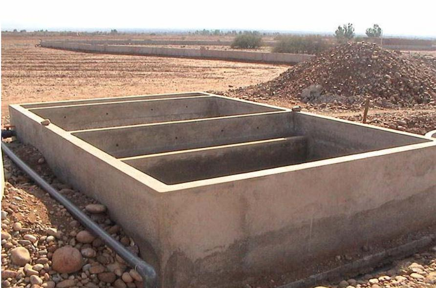
**Two-unit -horizontal-vertical gravel filter**
