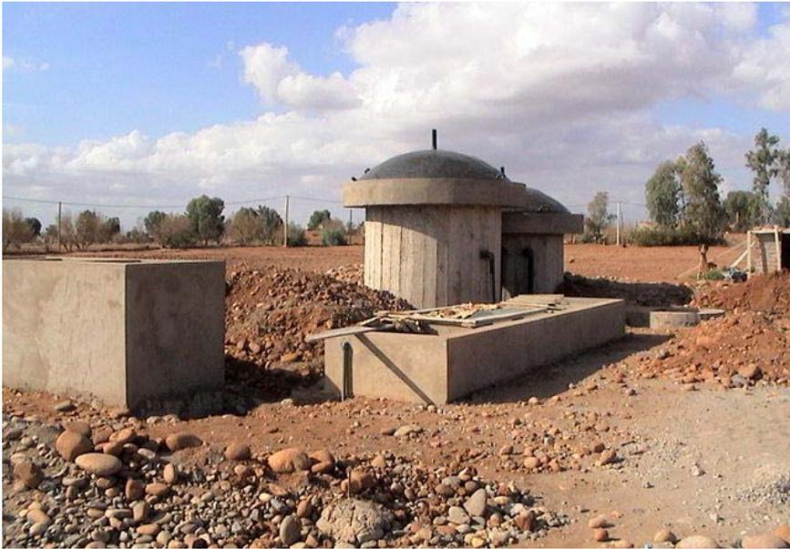
**Reactors, Settler and sludge drying beds**
