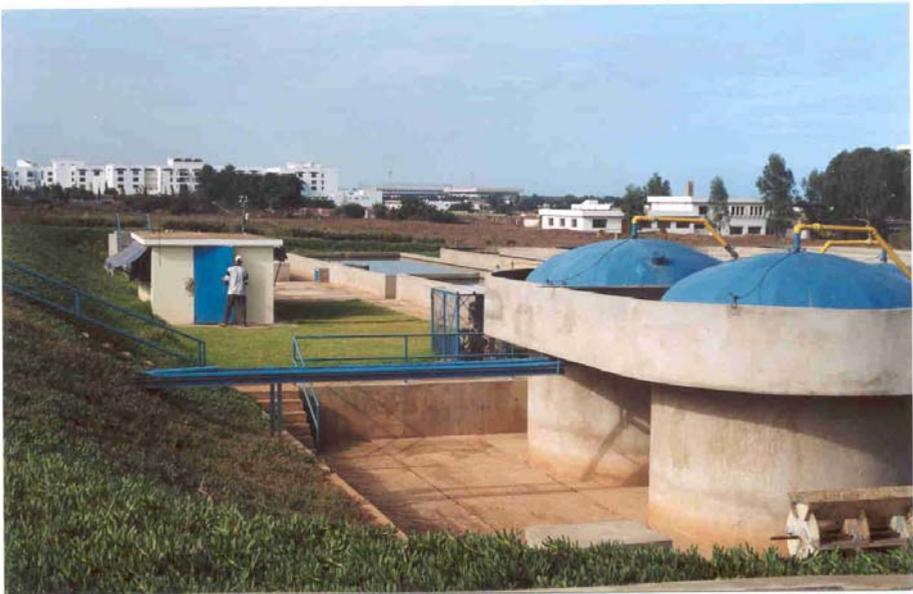
**Anaerobic reactors and maturation ponds**
