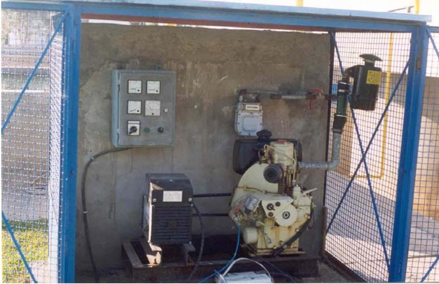
**Diesel-biogas combined generator**
