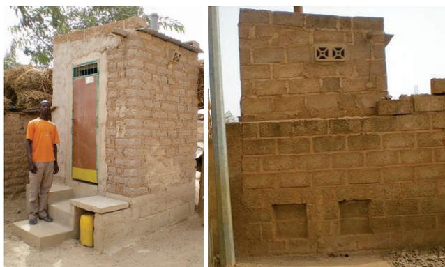
**Figure 2.** Left: Outdoor UDDT with stairs in Ouagadougou, Burkina Faso (photo: A. Fall, 2009). Right: Rear view of a similar UDDT in Ouagadougou showing the dehydration vault access doors (photo: S. Tapsoba, 2009).
