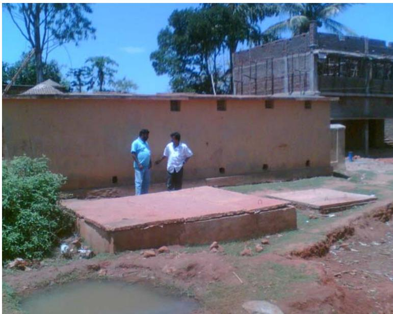
Figure 13 : Septic tank and soak pit
