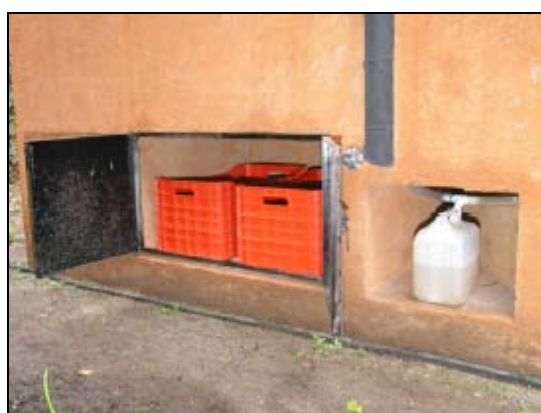
Figure 2-5: Dehydrating chamber with two faeces containers and urine collection – low cost version (UNESCO-IHP and GTZ, 2006)
