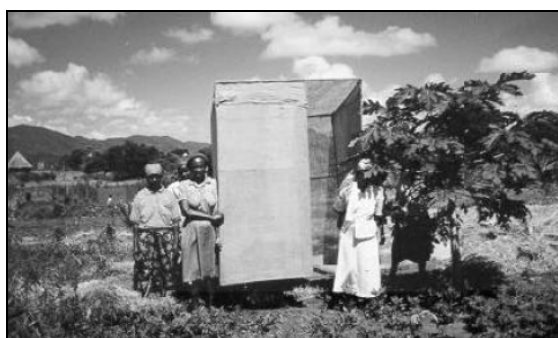
Figure 2-6: Arborloo - leave the contents, move the “loo” 10 and plant a tree (Esrey et al., 2001)
