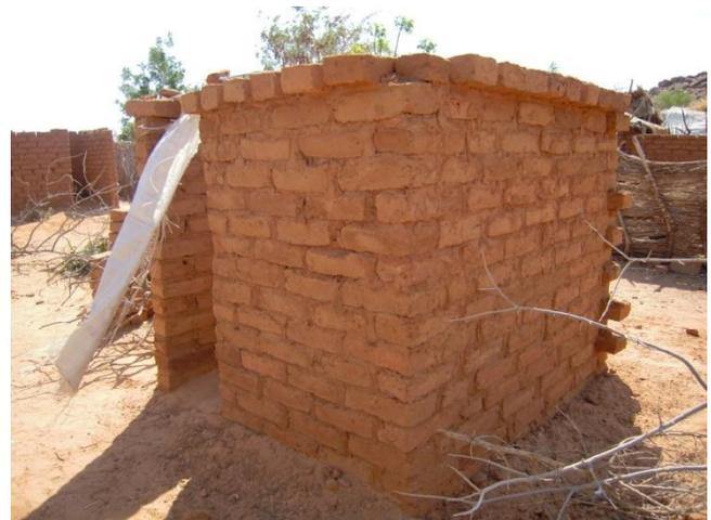
**Fig. 4:** Superstructure of a double pit latrine. **Is this the material usually used for the superstructure? Fig. 7 indicates a much simpler version. Do the pit latrines not have a roof? Why? What about privacy or similar issues?** (Source: J. Patinet (2009) Groupe URD).
