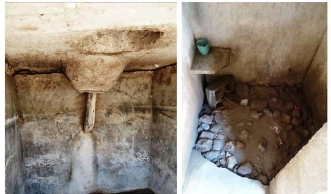
**Fig. 9:** Situation 8 years after construction: Left: walls of faeces vault with deep cracks. Right: bathing cubicle's concrete floor is broken (source: A. Leitner, 2011).
