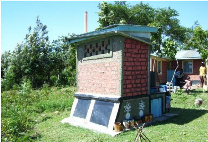
**Fig. 6:** Back view of household UDDT near Bungoma town in Western Province with two faeces vaults and ventilation pipe (source: Moses Wakala, GTZ-Kenya, Jan. 2010). Note: The inclination of faeces vault doors is not necessary for proper function – see Section 11. Moreover note the toilet is in relative close distance to house.
