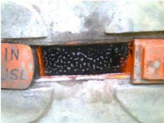
**Fig. 14** A urine pipe of a urine diversion squatting pans got blocked with ash at Muslim Primary School, Mumias. Faeces drop holes are covered with lids on the left and right in this photo (source: Laura Kraft, GTZ, June 2010).
