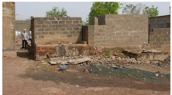
**Fig. 8:** Former desiccation (drying) chambers of UDDTs have been converted into pits to collect faeces and to be pumped empty when full (source: Stefan Hofstetter, March 2009).
