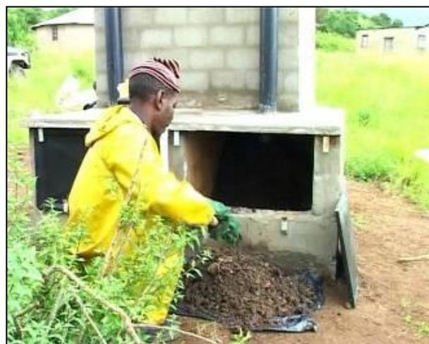
**Fig.14:** Emptying a UDDT faeces chamber (source: EWS.).
