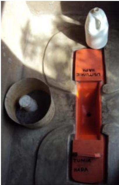
Fig. 7 Plastic urine diversion squatting pan with concrete footsteps inside a UDDT. Urine is collected in the centre; the two lids are covering the two faeces vaults (source: Laura Kraft, GTZ, June 2010).
