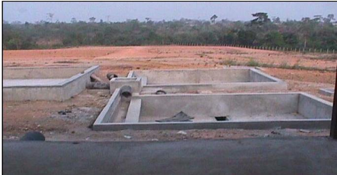
Fig. 4: Faecal sludge drying beds (source: Olufunke Cofie, 2002).
