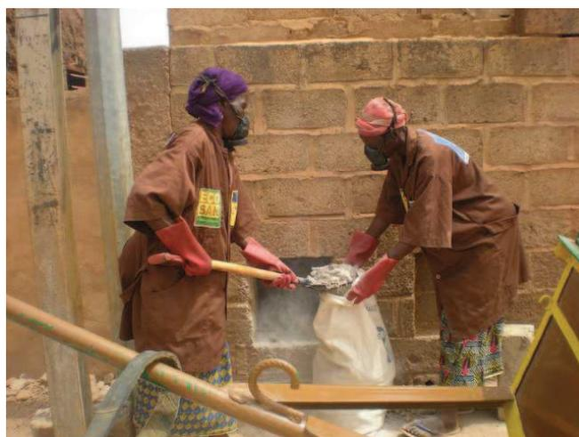
Figure 1: Two staff members from a service provider are emptying the faeces vaults of household UDDTs in Ouagadougou, Burkina Faso (source: S. Tapsoba, 2009)<sup>1</sup>.
