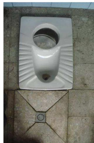
**Fig. 9:** Urine diversion squatting pans with a third outlet in the front for anal cleansing with water (source: K. Sintayehu, 2010).
