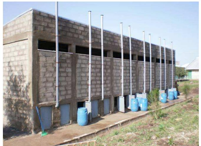
**Fig. 8:** Back view of the UDDT block showing vent pipes and blue doors to faeces vaults (source: K. Sintayehu, 2010). Note the blue bins should be inside of the faeces vaults.
