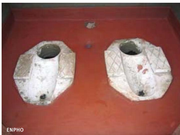
these pans in general. The one major problem area was the connection between the urine pipe and pan, as with the combined pan. Many toilets surveyed were found to leak at this point.
