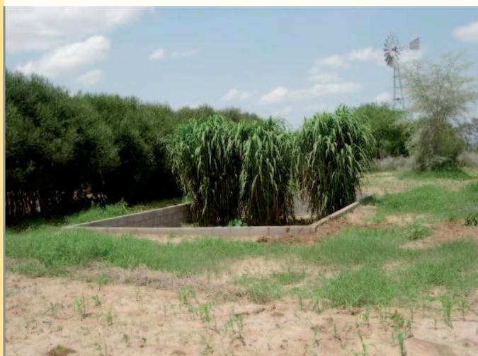
Picture 2: Horizontal flow CW system in Kanawat Health Centre.
