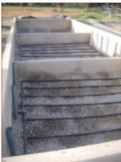
Figure 7. Tertiary VF Sand Filter Cross Photo (2011)
