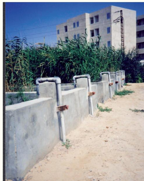
Figure 3: Effluent sampling points at the 6 1st stage HSSF beds
