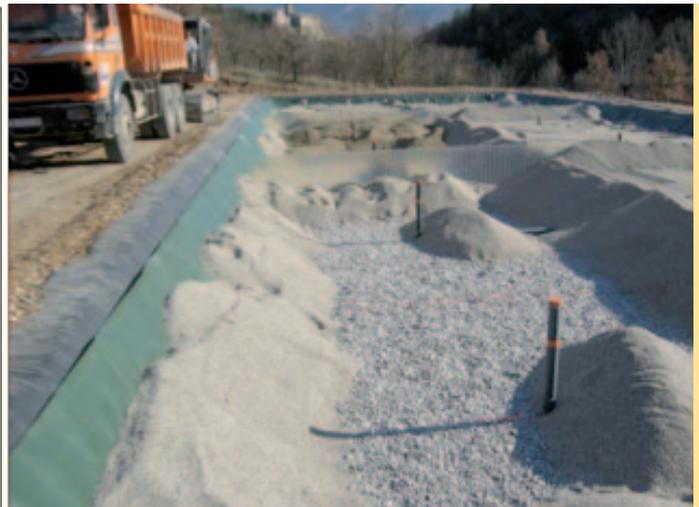
Figure 5: Putting in filtering materials on the 1st stage (Epur Nature)
