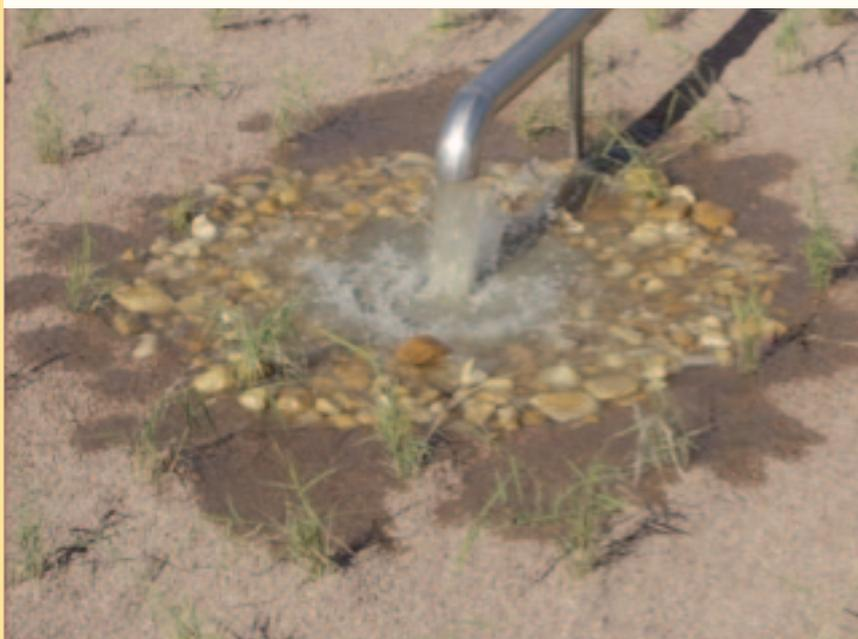
Figure 6: First stage feeding device (Epur Nature)
