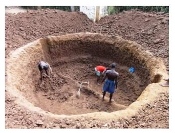
Figure 1: Excavations for a biogas digester in Livingstone, Zambia at a project of the Devolution Trust Fund (DTF) (source: P. Feiereisen, 2011)
