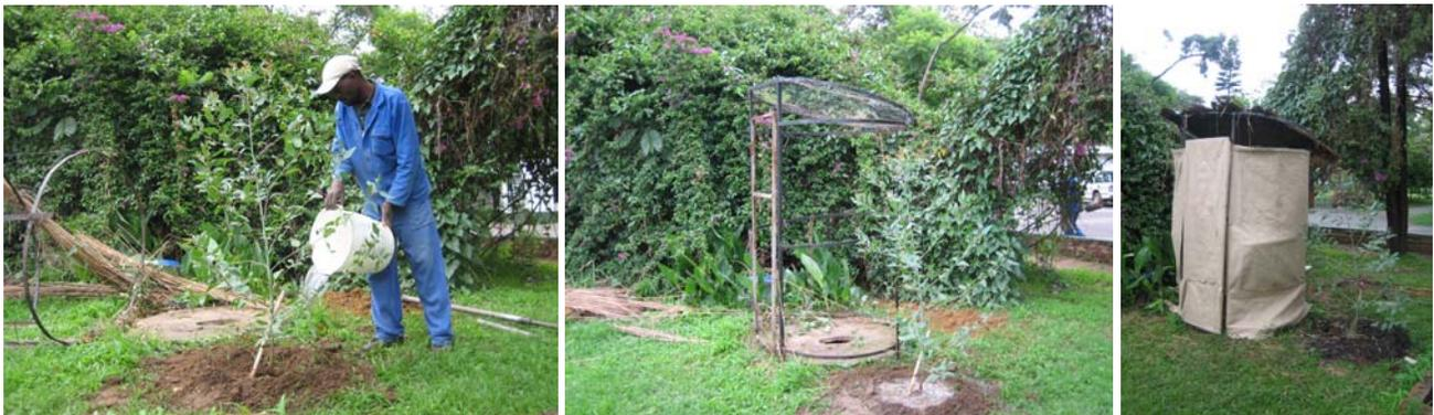
The planted tree was watered. The wall covers of the steel frame portable structure were rebuilt in hessian material. The pit was protected by a concrete ring beam only with faeces in direct contact with the soil of the pit walls.
