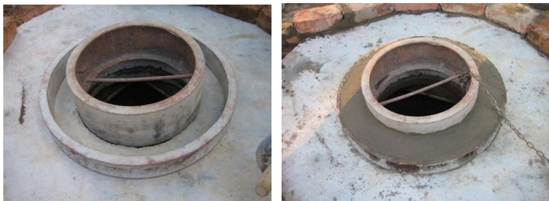
**The annular space between the shuttering is filled with a strong concrete mix of 3 parts river sand and one part PC 15 cement with a ring of steel wire half way up the collar. This is left to start hardening and the shuttering is removed some hours later.**
