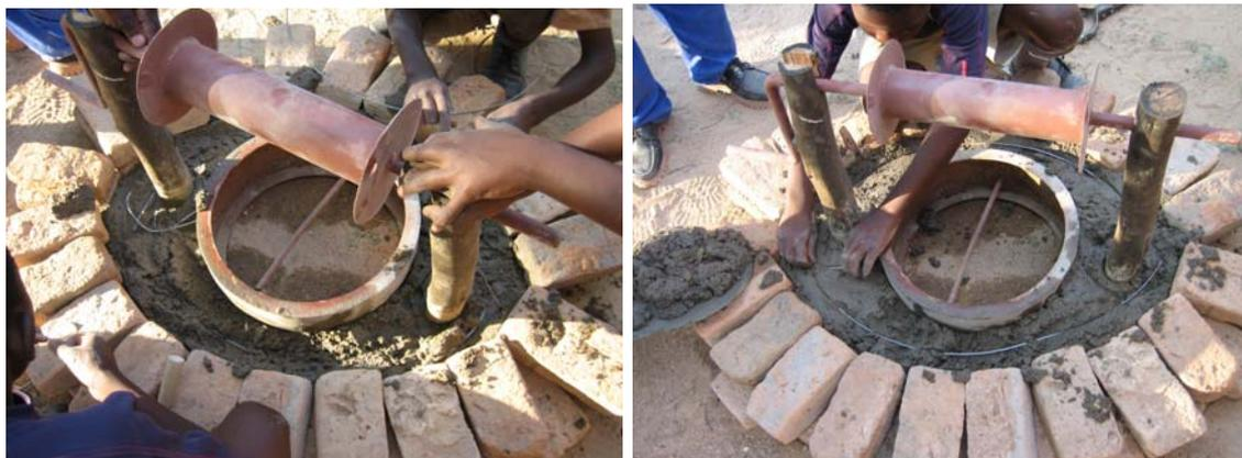
The concrete is added to the mould with plenty of reinforcing wire
