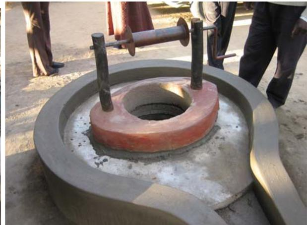
**The windlass system is mounted around the well access hole leaving enough room on either side to allow water to drain away down into the run off system. A further layer of mortar is added to the well slab and finishing touches are made all over the well to make it neat, strong and tidy. The new upgraded family well can then be put to use.**
