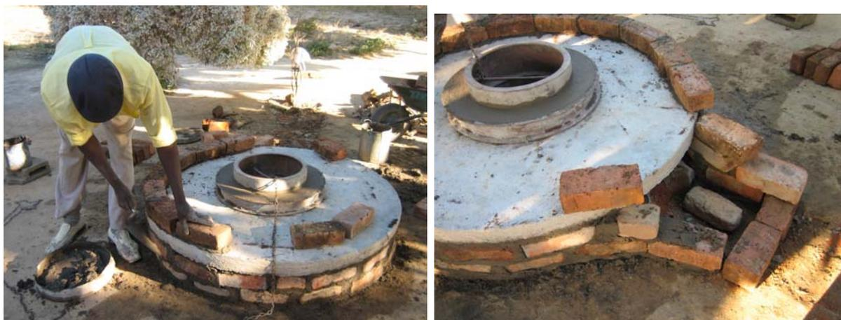
**The larger slab is supported by layers of bricks built beneath it as shown in the photos. This lower layer of bricks is extended forwards to support the water run-off channel which will be built later.**
