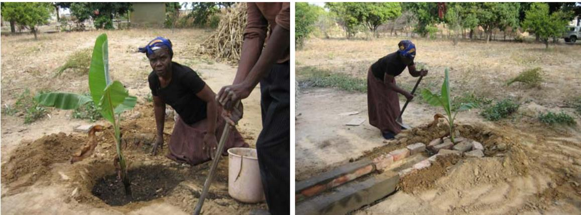
**Water flowing down the run-off should drain into a seepage area. This is best made into a hole filled with humus like soil and planted with a suitable tree like a banana, which can absorb the water and also produce valuable fruit.**
