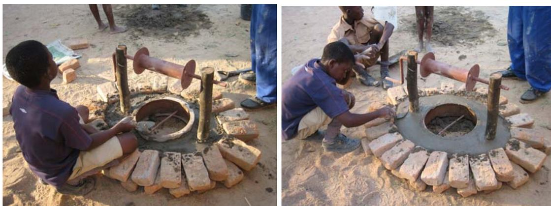
The mould is filled up so the concrete is at least 15cm deep
