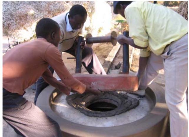
**Once the raised collar system was been removed and the well cover cleaned down some strong cement mortar is laid down around the well access hole for the windlass system to lay in.**
