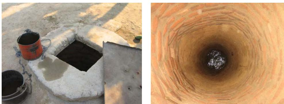
**Views of a simple poorly protected well head and down the well chamber**
