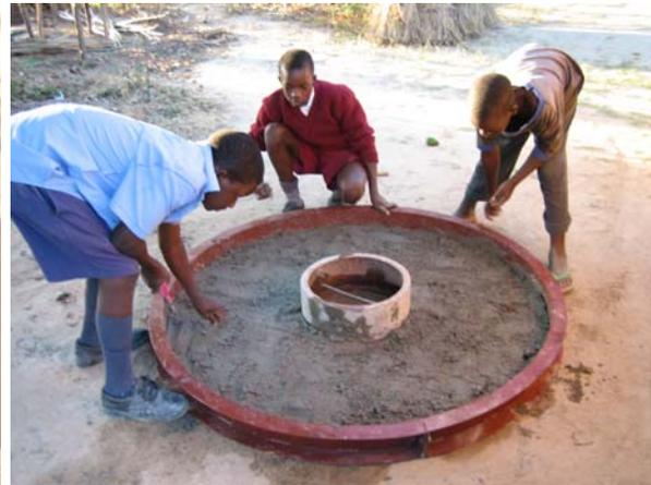
**The shuttering is laid down on level ground overlaid by sand which is wetted. Half the concrete mix is added and levelled off.**
