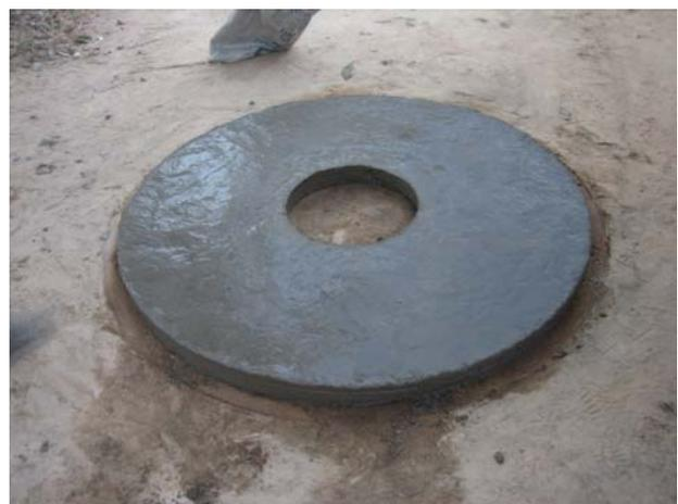
**The 3mm steel reinforcing wires are added in a grid formation. Then the second half of the concrete mix added and smoothed off. The shuttering is then removed. This is allowed to harden overnight and then kept wet under a plastic sheet or wet sand for a week before moving.**
