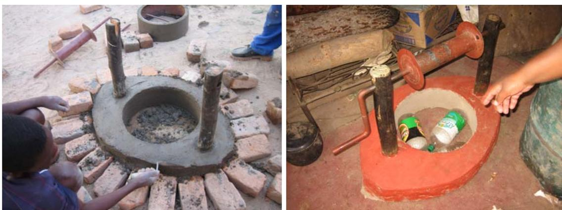
The concrete is allowed to harden a little. Then central round mould is removed followed by the windlass. The concrete work can be shaped up to be neat. The concrete anchor, supporting the two windlass support poles is left to cure for at least 2 weeks and is kept wet at all times. In the future this concrete anchor will be put to the test as the windlass is used.
