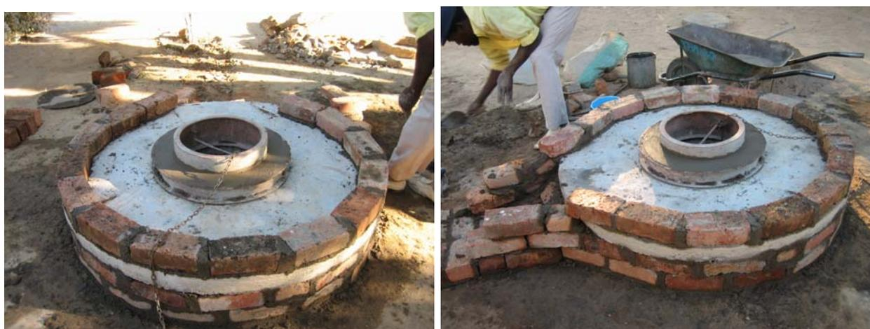
**Bricks being laid so that drained water will flow into the water channel.**
