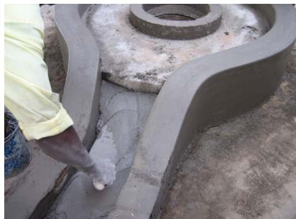
**The strong mortar work extends down the slope leading from the slab to the water run-off channel.**
