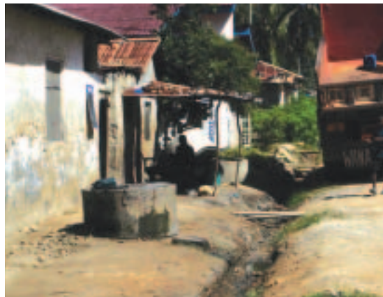
This is a protected well. But is the water safe, next to an open sewer?
