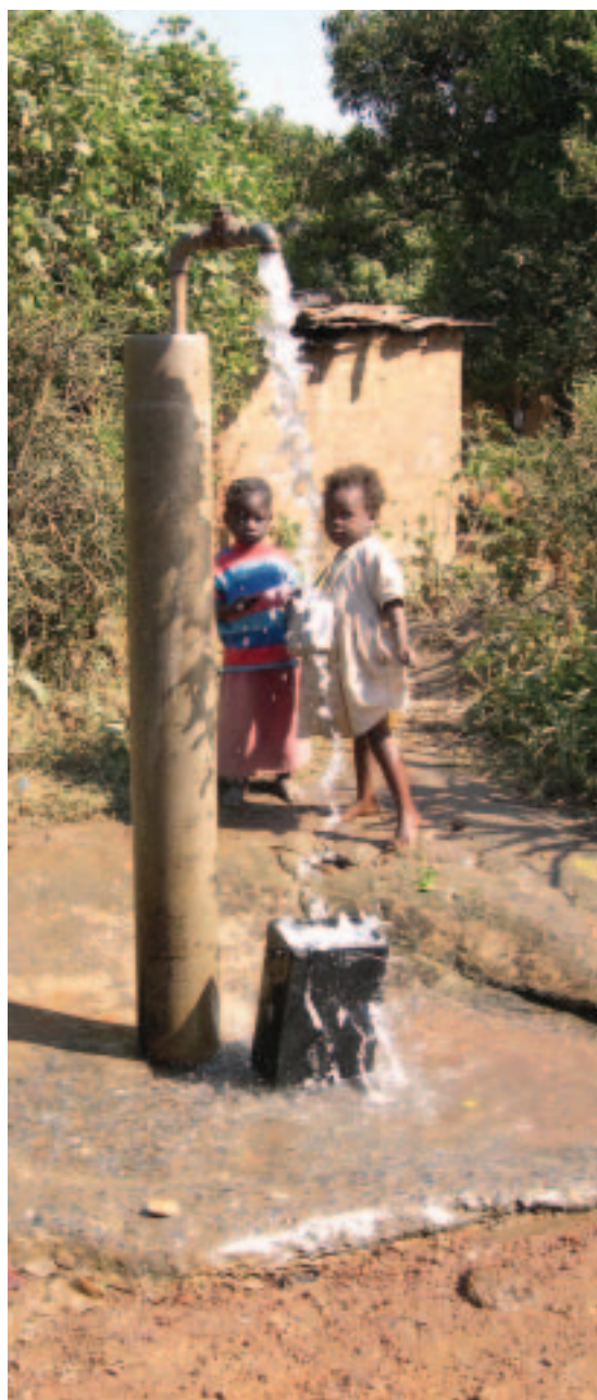
Standpipe without valve in Zambia.
