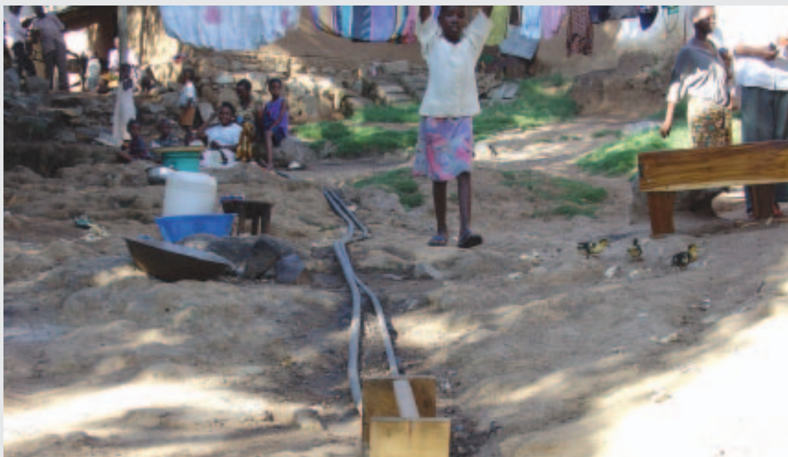
An illegal connection brings water into an urban neighbourhood.
