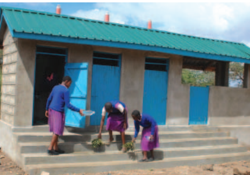
Ventilated improved latrines built above ground level to avoid potential flooding. Photo by Sustainability Africa.
