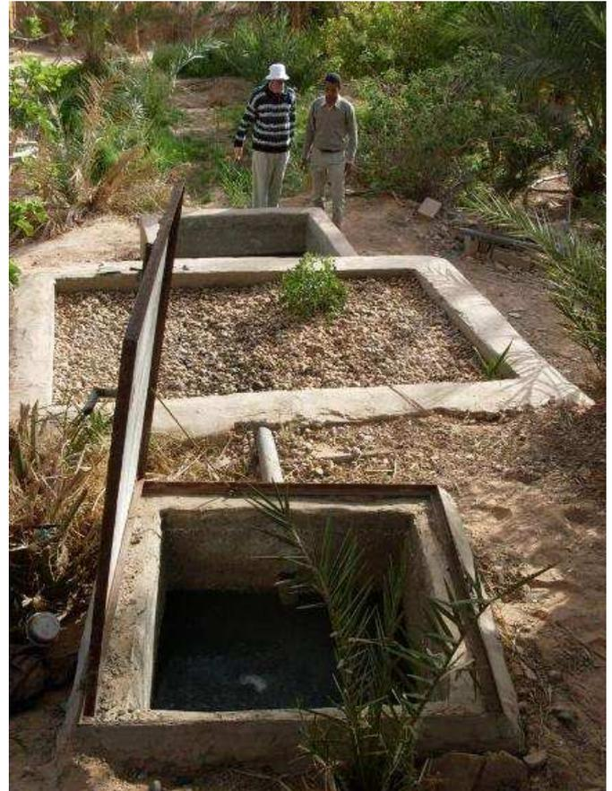
**Fig. 8:** The grease trap /settlement basin, filter and storage tank for the irrigation of the vegetable garden and the house of Mr. Boussouri (garden visible in the background) (source: AHT GROUP AG, 2011).
