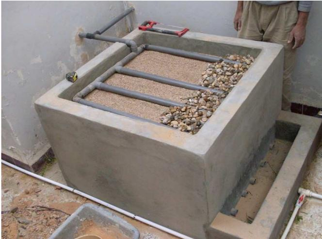
**Fig. 7:** Settled greywater is distributed across the surface of the filter medium using a series of perforated pipes (source: AHT GROUP AG, 2011)
