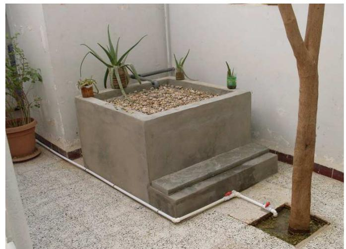
**Fig. 10:** The rebuilt greywater filter at the project offices in Béni Abbès (source: AHT GROUP AG, 2011).
