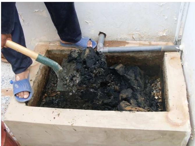
**Fig. 9:** Excavation of the completely clogged filter media in the original (source: AHT GROUP AG, 2011).
