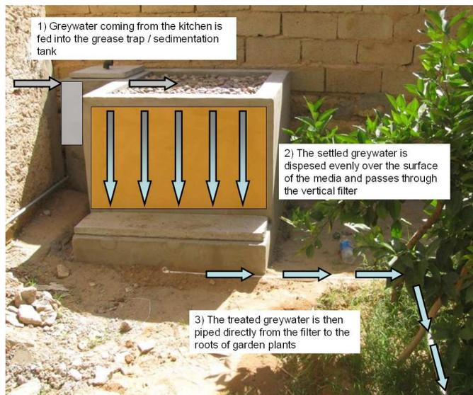
Fig. 5: Schematic of the greywater flow from the kitchen sinks, through the treatment system, to the garden plants.
