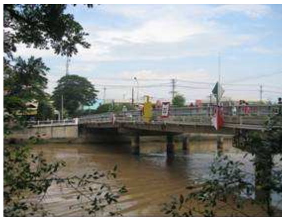
Figure 4-5 Long Binh 1st Bridge :as surface water
