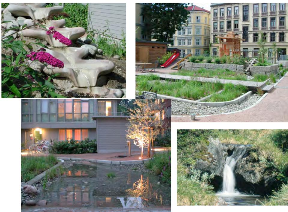
*Fig. 2. The klosterenga greywater treatment system. Upper right; the wetland in the foreground the biofilter is underneath the playground behind the stonewall. Upper left; Flowforms. Lower left the effluent is exposed in a shallow pond. Discharge to a local stream is possible is the stream was reopened.*
