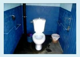
This school toilet was modified to include a toilet seat and hand rails to enable greater access (left photo). However, the cubicle was too narrow to allow a wheelchair user to turn; this meant Andry had to turn herself around using the rails for support. The support rails were also too high. The re-modelled version is 1.5 metres wide which allows Andry to turn in her wheelchair inside the cubicle. The lower rails allow a person to transfer themselves using one rail (right photo).
