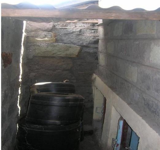
**Figure 9** The rear of the UDDT showing vault doors and a shade for temporary storing the faeces for further drying before utilisation/disposal.
