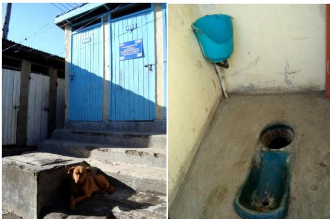
**Figure 10** On the left, the old pit-latrines used by the tenants are located next to the UDDT facility with greywater settling chamber in front. Right: Only one cubical and one urinal of the UDDT are currently used by the landlord and his family (L. Kraft, May 2011)
