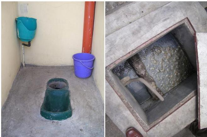
**Figure 6** On the left: Inside the single vault UDDT showing the urine diversion pedestal, men's urinal and a bucket for storing ash. On the right: greywater settling chamber
