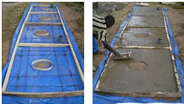
**Photograph 10 Casting Fossa alterna slabs**
