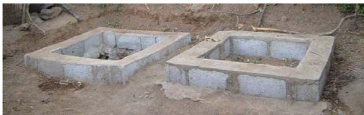
**Photograph 9 Fossa alterna ring beams**
