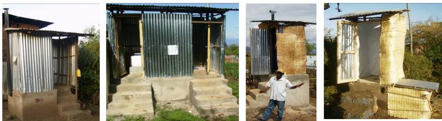
**Photograph 7 some of the UDDTs constructed with different material**
