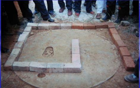
The use of brick extended to the construction of the vent pipe. Whilst not as effective as the smooth walled steel, PVC or asbestos pipes, it was cheaper and could be built on site. This unit was built more than any other
