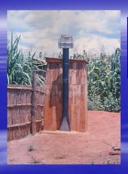
Flies were counted in a trap fitted at the top of the pipe. This showed that if the toilet house was dark enough, almost every fly would travel up the pipe rather than out through the squat hole.
