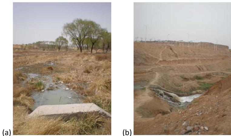
**Figures 4-1a and 1b.** Discharge outfalls for (a) EETP treated greywater and (b) Dongsheng STP treated wastewater.
