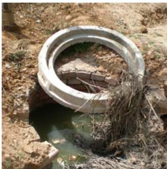
**Figure 7-18.** Overflowing treated greywater effluent from a damaged manhole. [A. Flores, taken 22 April 2009.]
