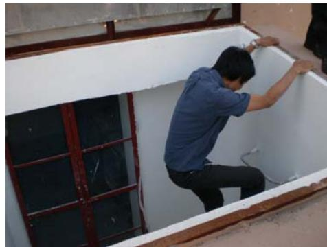
**Figures 4-4a and 4b.** Views of the covered pit access to the basements at the EETP. Bins are moved in and out of the basements using a hoist attached to the bin collection truck. [A. Flores, taken 5 September 2007.]
