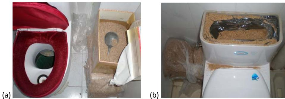
**Figures 4-3a and 3b.** Sawdust use in the UDD toilets. (a) Example of a well-maintained UDD toilet with a sliding plate mechanism. Note that the household is using a box instead of the dispenser. (b) Example of the mess that can be caused by sawdust. [A. Flores, taken September 2007.]
