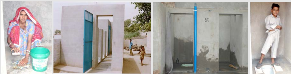
Figure 12: A combined model of simple pour-flush latrine and a separate wash room was jointly developed with the target groups in a KfW supported sanitation project in Rajasthan. (Source: KfW)
