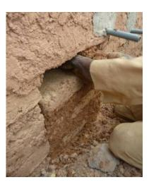
**2.** Close off the vaults with bricks and light mortar to avoid that water and flies can enter.
