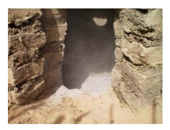
**1.** Add ash or straw on the bottom of the vault to absorb humidity and avoid that the faeces sticks to the bottom.
