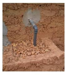
**4.** Make sure that the anal cleansing water enters the small soak away.
