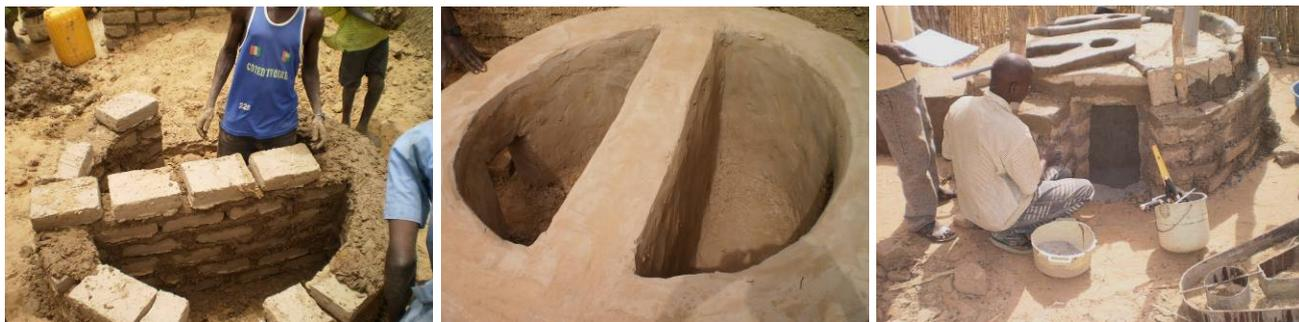
The vaults are constructed off the ground. The slab is placed on the vaults. When the vaults are off the ground, the rain cannot inundate them and the sun can heat the walls and help drying out the faeces.
