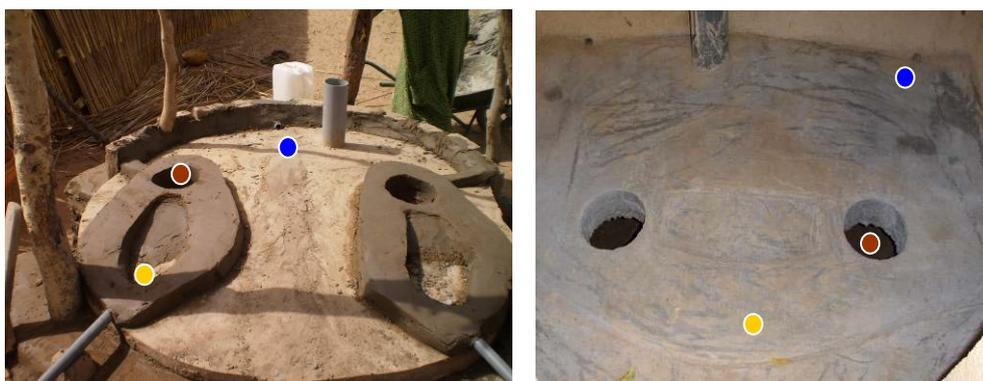
The urine separation on the slab can be done in different ways. The anal cleansing water is drained separately from the cabin.
