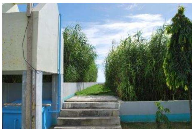
Figure 27. Subsurface flow CW in Bayawan city, Philippines. The path in the middle separates the VFB and the HFB (photo by J. Boorsma, 2009; project supported by GIZ)<sup>24</sup>.
