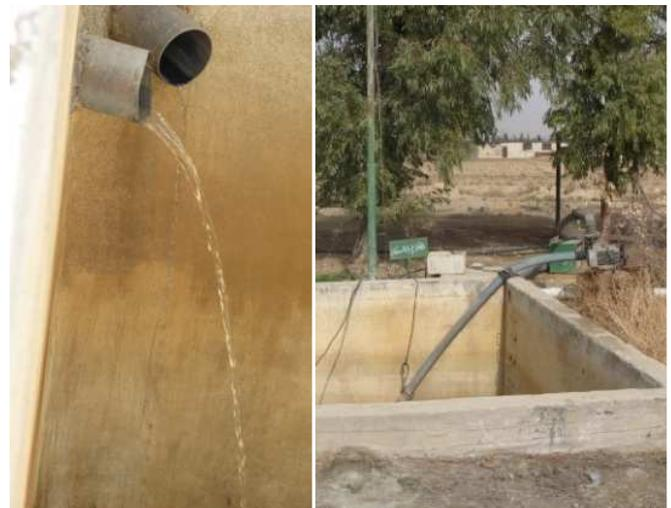
Figure 3. The treated effluent (left) of the vertical flow constructed wetland in Haran Al-Awamied, Syria, is collected in this storage tank (right) before its reuse for irrigation in agriculture (photos by E. von Muench, 2009; project supported by GIZ).
