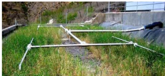
Figure 26. Distribution pipes for raw wastewater in first stage (VFB) in French System in Albondón, Spain (photo by T. Burkard, 2007).
