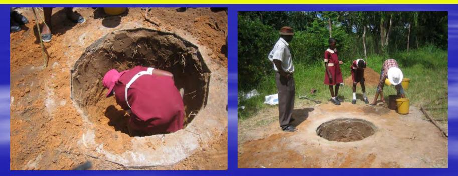
Moving the slab on to the ring beam. Since neither the slab or ring beam are perfectly flat a layer of weak cement mortar or damp termite soil is laid on the ring beam.
