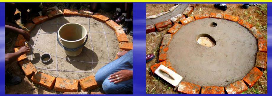
Dig the pit and line with bricks In this case the toilet is being made by school children and the pit is dug down to only one metre deep. Normally a pit will be dug down to 2 or more metres deep. Fired bricks are gathered.
