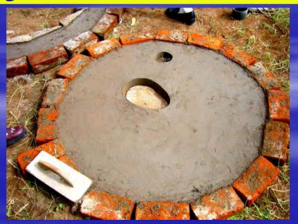
The slab is now curing Now we find the place where we will build the toilet, clean up and level the area and mark the spot for the ring beam
