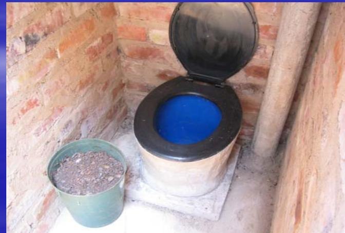
*This new generation of toilets in which composting is encouraged in alternating pits may solve some of the existing problems of pit latrines.*
