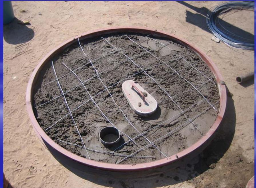
*The three concrete pieces are left to harden and cure for several days. The soil within one ring beam which will be used for the toilet is now dug down to 1.5m with the second dug down to 0.3m.*
