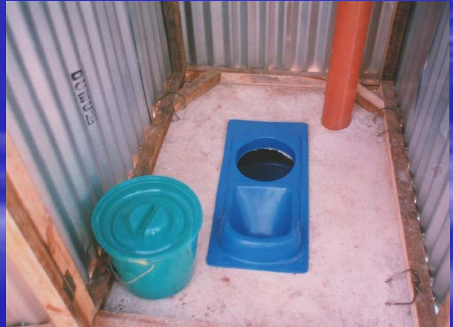
*Most urine diverting toilets use two alternating vaults to retain the faeces but it is possible to use a single vault*
