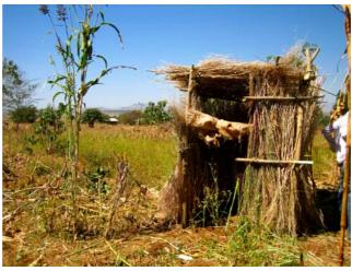
The fifth post is added in between the two front posts and half of this is also filled with walling material. The opening is for the door which can be covered with a cloth handing down from the upper beam. A simple door on rubber hinges (car tyre etc) can also be added.
