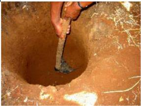
The larger the diameter of the hole and the deeper the pit, the longer the pit will last. Some people may prefer smaller holes if they want to plant more trees, but this means moving the slab and "toilet house" more often. The larger the pit is, the longer it will take to fill up and moving the slab and house does not need to take place so often.
