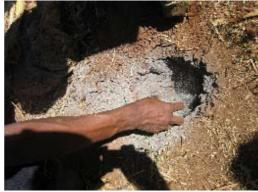
The corner posts being dug. Ash being added to the holes before poles inserted. Soil is rammed in the holes around posts to secure.
