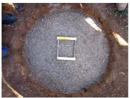
Wires are also cut. The wire can be 2mm or 2.5mm thick. 4 wires are cut to 0.7m and 4 to 0.6m. A frame for the squat hole is then made of wood. This is 20cm by 15cm. These parts are placed in the hole to test for size as shown in the photos.
