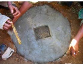
The wooden squat hole frame is removed and the edges of the hole are made neat with a trowel. Wire handles can be added, but with small slabs they are unnecessary. The slab is made neat and smooth using the steel trowel.
