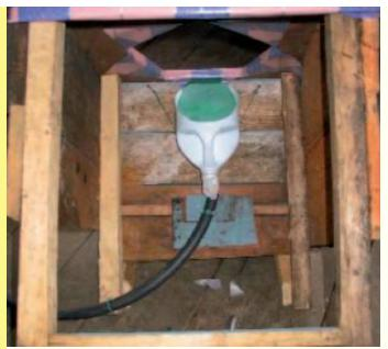
Figure 3: View inside the toilet, showing solidly fixed 1" black hose and easily removable white funnel
