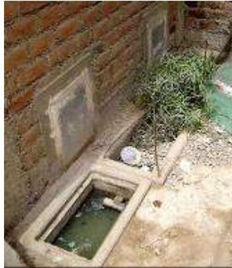
Figure 2: Until 2007 UDDT in Lima always mixed grey water with urine, but the infiltration often didn't work properly.
