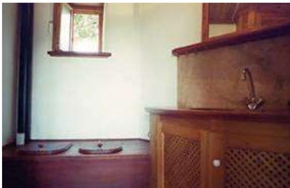
Figure 10: Dry toilet integrated into a bathroom.
