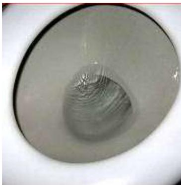
Figure 7: Water loss due to malfunctioning of water valves.
