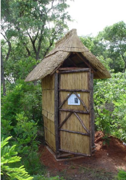
Figure 3-1: Simple compost toilet built on rectangular slab
