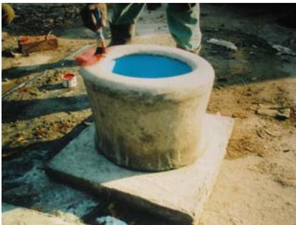
Figure 5-5: Painting the concrete pedestal
