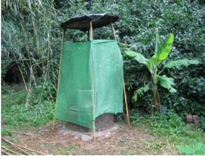
Figure 7-7: Structure around upgraded toilet
