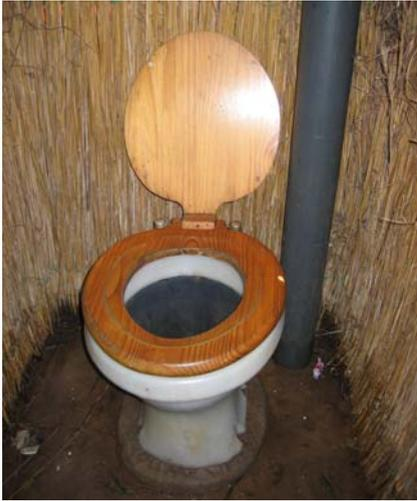
Figure 7-11: *Fossa alterna* upgraded with a non urine-diverting pedestal
