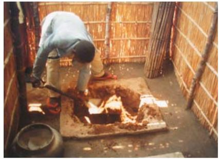
Figure 4-22: Excavating the humus from the pit
