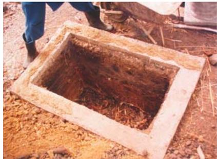
Figure 4-12: Completed *Fossa alterna* pit
