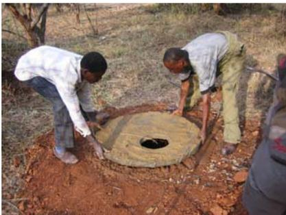
Figure 3-49: Slab placed over ring beam
