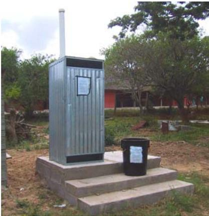
Figure 4-27: *Fossa alternata* with a metal structure
