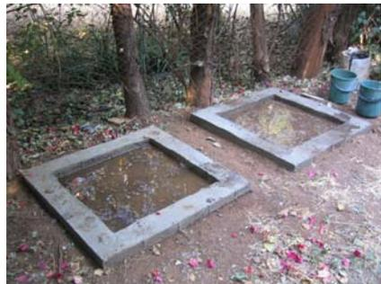
Figure 6-48: Cured ring beams
