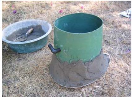
Figure 6-20: Concrete added half-way up the bucket
