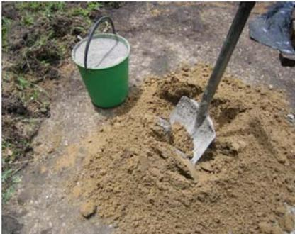
Figure 3-24: Mixing the cement and river sand
