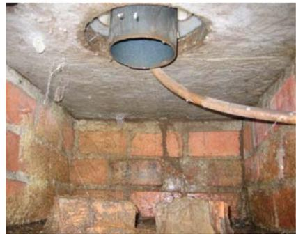
Figure 7-14: Urine pipe located below the slab
