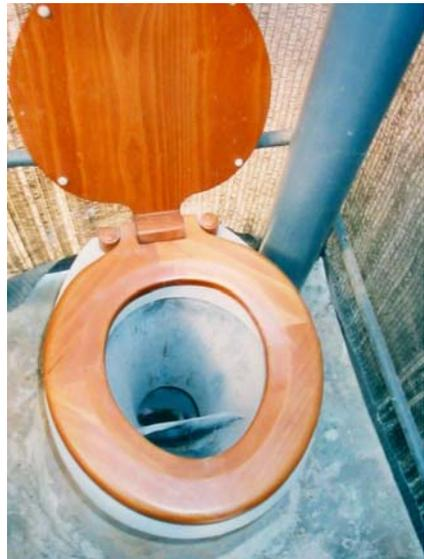
Figure 6-36: Top-view of the a urine-diverting pedestal
