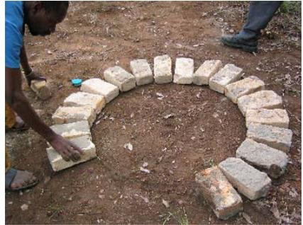
Figure 3-10: Forming the brick ring beam
