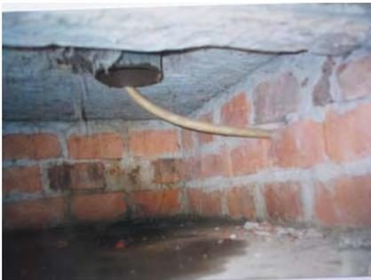
Figure 6-37: Plastic pipe carries urine from the urine-diverting pedestal
