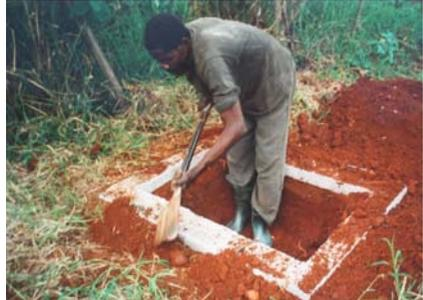
Figure 4-10: Digging the pit for the *Fossa alterna*
