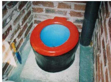
Figure 5-6: Finished concrete pedestal
