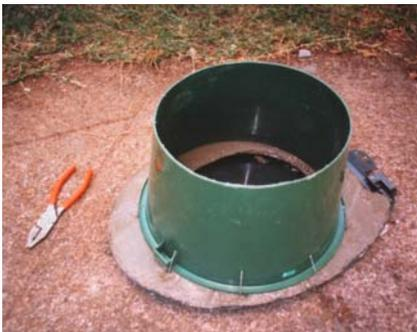
Figure 5-9: Plastic bucket placed over toilet seat
