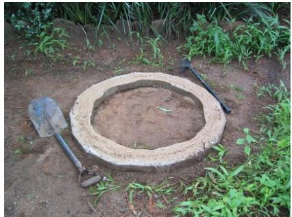
Figure 3-17: Completed ring beam
