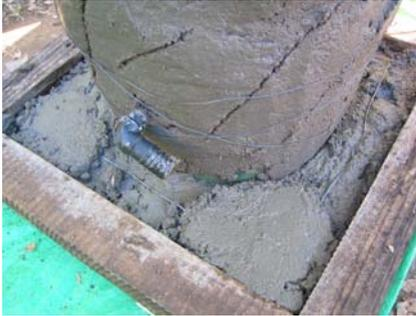
Figure 6-23: Wire added for reinforcement
