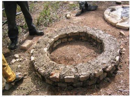
Figure 3-12: Completed brick ring beam
