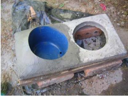
Figure 6-33: Top-view of a urine-diverting squat toilet
