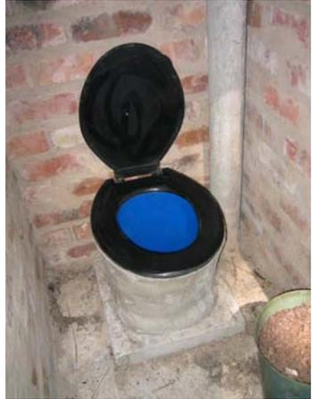
Figure 5-12: Completed low cost pedestal with plastic seat
