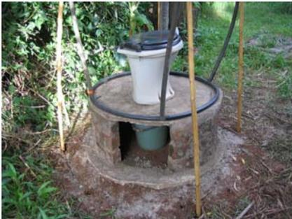
Figure 7-5: Slab and pedestal fitted on built-up base
