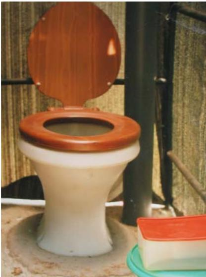
Figure 6-35: Urine-diverting pedestal with a handsome wooden seat
