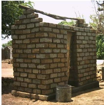
Figure 4-28: Brick double pit composting toilet
