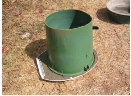
Figure 6-18: Bucket placed onto the toilet seat
