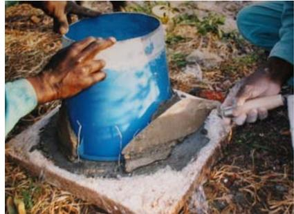
Figure 5-4: Building up the sides of the bucket
