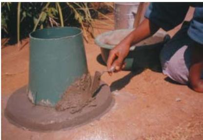
Figure 5-1: Construction of the very low cost pedestal
