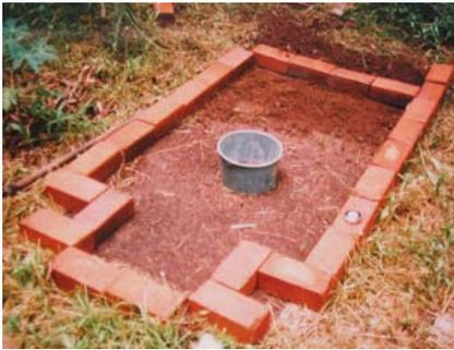
Figure 6-1: The brick mould for the base slab
