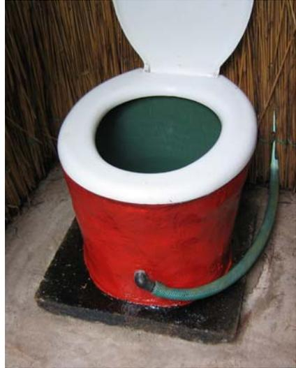
Figure 8-2: Urine-diverting pedestal
