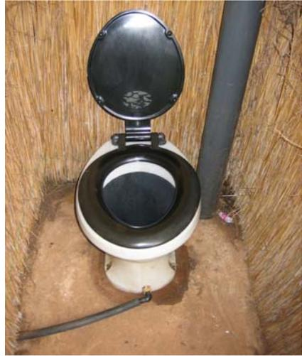
Figure 7-12: *Fossa alterna* upgraded with a urine-diverting pedestal
