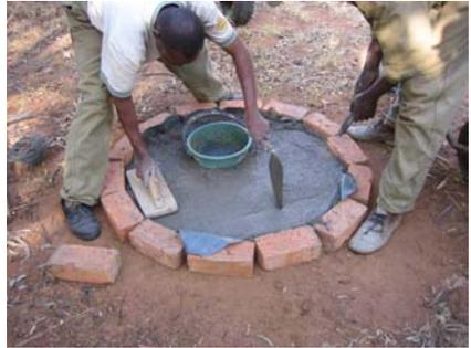
Figure 3-42: Levelling-off the concrete mix
