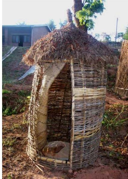
Figure 3-2: Toilet house built over a round slab in Malawi
