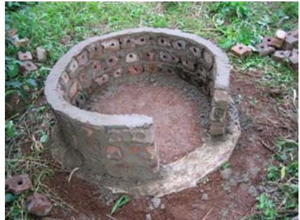
Figure 7-4: Brick wall built-up on ring beam
