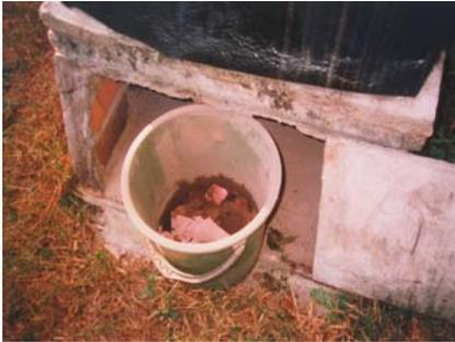
Figure 6-43: Removal of bucket of faeces
