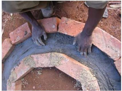
Figure 3-44: Addition of wire for reinforcement
