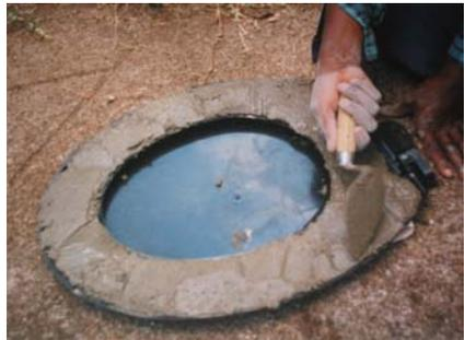
Figure 5-8: Plastic toilet seat filled with strong concrete
