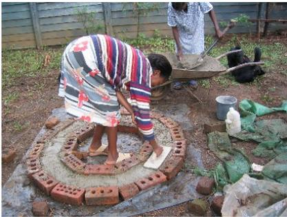
Figure 3-16: Levelling off the concrete
