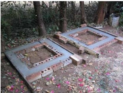
Figure 6-47: Casting ring beams
