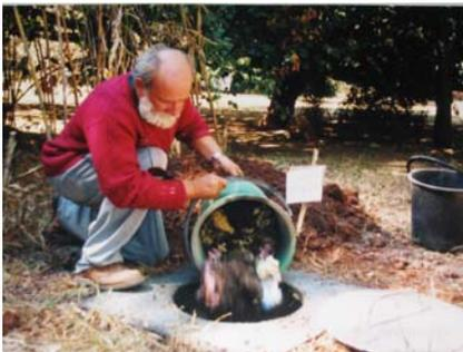
Figure 6-45: Emptying faeces into a small shallow pit
