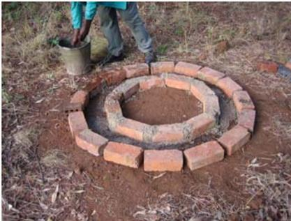
Figure 3-43: Ring beam mould using bricks
