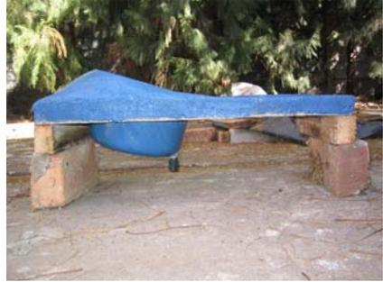
Figure 6-34: Side-view of a urine-diverting squat toilet
