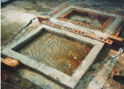
Figure 4-9: Ring beam mould using bricks
