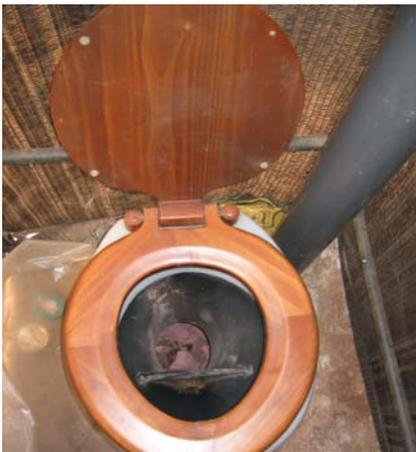
Figure 6-57: Cleaned urine-diverting toilet
