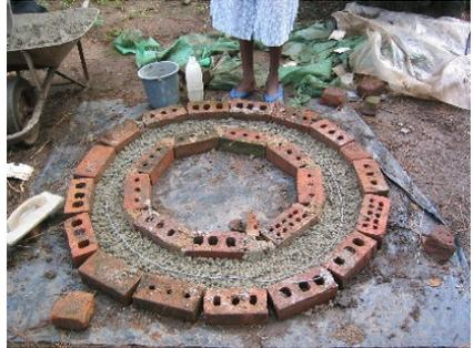
Figure 3-15: Cement and wire reinforcement added to mould
