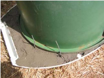
Figure 6-19: Bent wire added around the bucket
