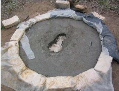
Figure 3-9: Mould after removal of squat hole insert
