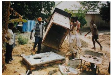
Figure 7-10: *Fossa alterna* built on a rectangular slab
