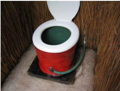
Figure 6-31: Urine-diverting pedestal installed
