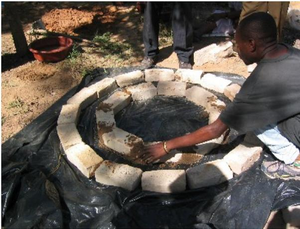
Figure 3-13: Brick mould on top of plastic sheet
