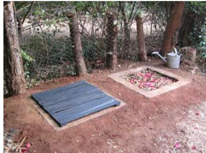
Figure 6-54: Active composting pit covered by wooden lid
