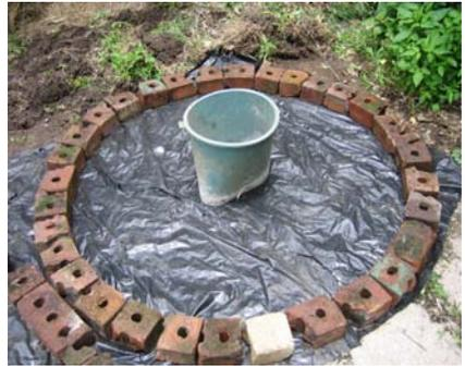
Figure 3-23: Shaped bucket to make the squat hole
