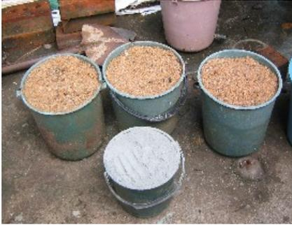
Figure 3-7: Measuring cement and river sand
