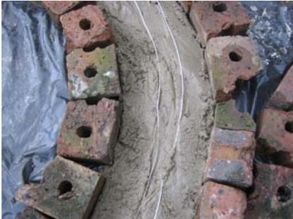
Figure 3-31: Wire reinforcement added
