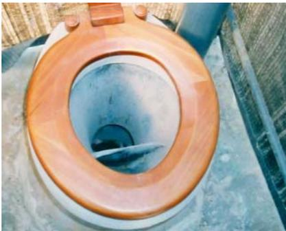
Figure 7-13: Urine-diverting pedestal mounted above the ground
