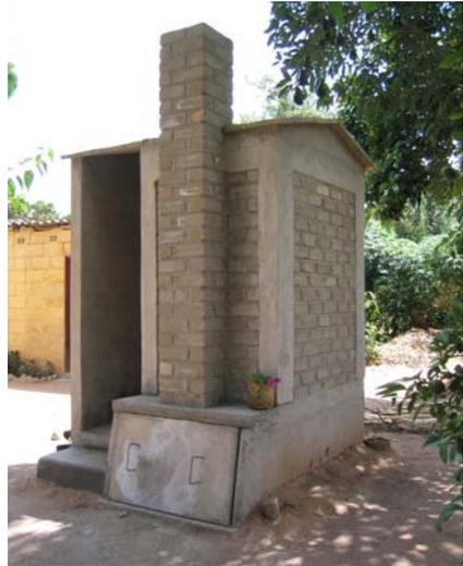
Figure 6-42: A brick single-vault urine-diverting toilet
