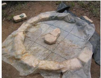
Figure 3-6: Sheet of plastic laid in the mould
