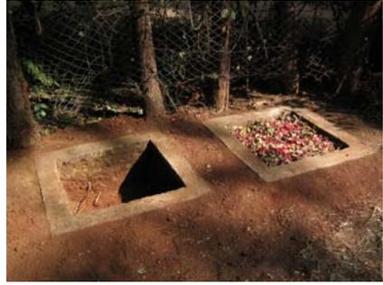
Figure 6-50: Twin pits ready for use with right-side pit filled with leaves
