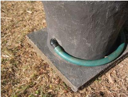
Figure 6-27: Urine outlet pipe attached
