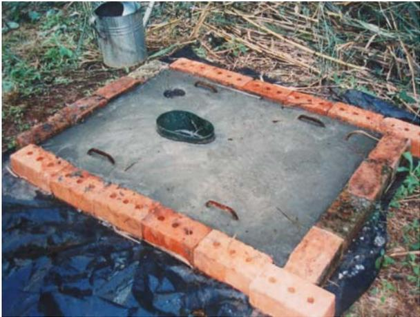
Figure 4-7: The completed slab inside the mould
