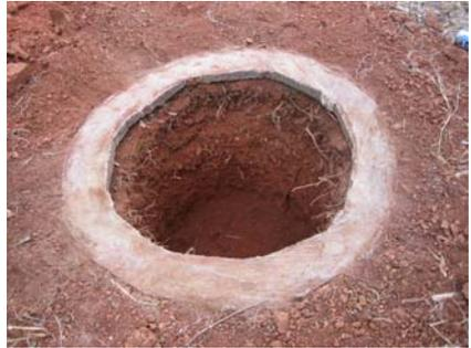
Figure 3-46: Pit dug inside ring beam
