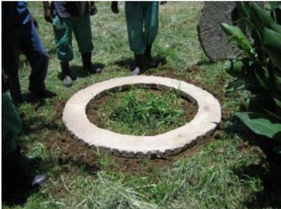
Figure 3-35: Placement of the concrete ring beam
