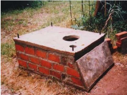
Figure 6-5: Fitting the vault access slab
