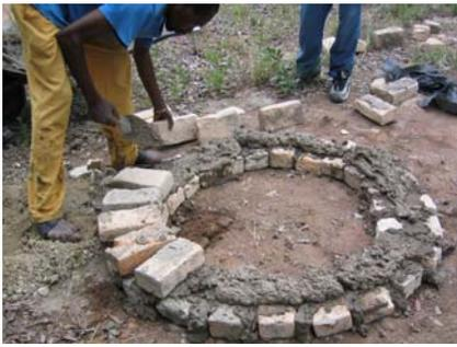
Figure 3-11: Adding the second layer of bricks with anthill mortar
