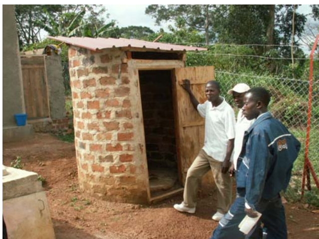
Team members take a transect walk through a community in Uganda to identify the level of latrine adoption and the variety of latrines used.
