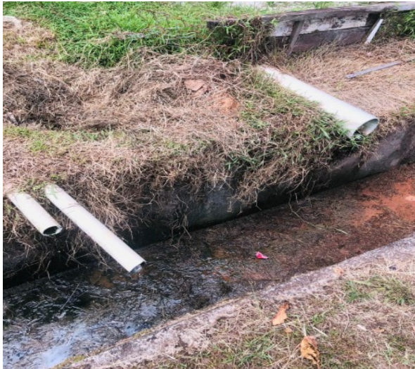
Figure 4: Pipe connected to Open Drain (Source: Rabicia/EPA./2022).
