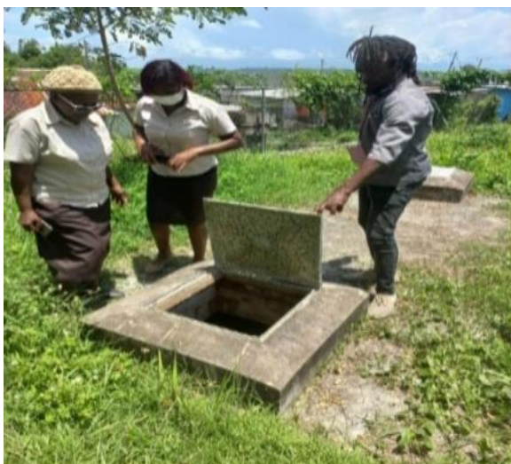
Figure 9: STs connected to soak pit (Source: Jodian/Org./2022).
