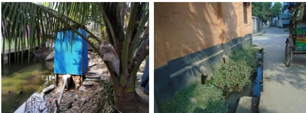
Figure 6: Containment technologies and their connections in Gaibandha. Left: Toilet pit connected to the nearby water body. Right: Toilet pipe connected to open drain. (Source: Feasibility study 2020-21/DPHE).
