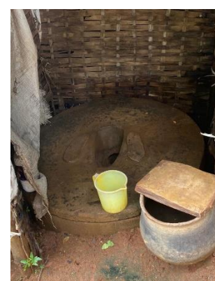
Figure 8: Pit latrine connected to unlined pit (Source: Dimple Behal/CSE).
