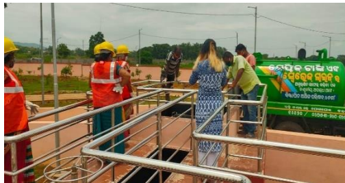
Figure 13: Discharging of FS at FSSTP (Source: Dimple Behal/CSE).
