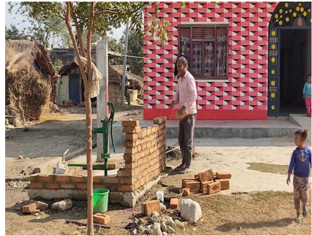
Figure 2: Construction work ongoing at Maya Ram's Uncle's hand pump (Source: UNICEF/Nepal)
